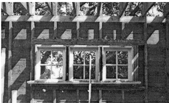
Figure 1. Walls of a wood-frame house built in 1919 at the University of Saskatchewan were filled with CFI in 1926 and opened in 1975. Inspection showed no traces of moisture and no damage.
