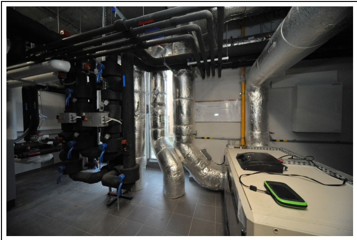
Figure 3. Mechanical room (CW1), reflective jackets on pipes from wall air intake and EAHX.
