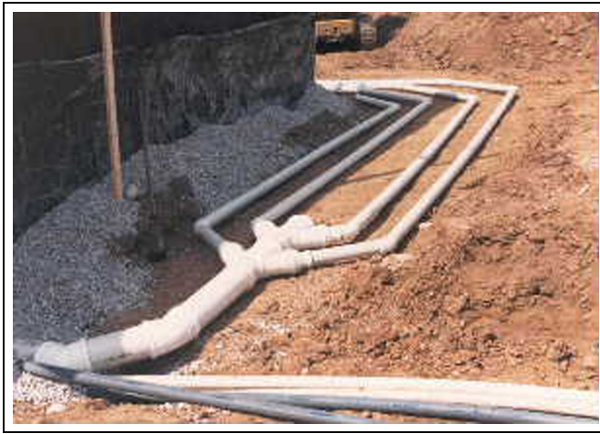
Figure 1. EAHX that is placed next to the drainage pipe.
